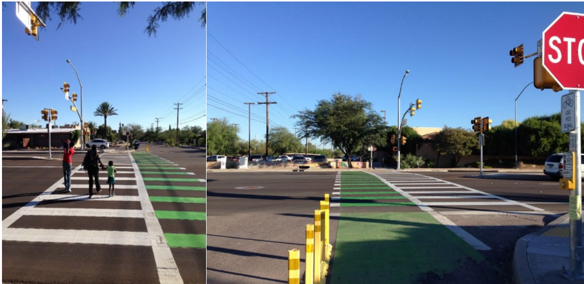
One of the first BikeHAWKs serving Pima Community College and Medical/Social Services Facility at W. Speedway and N. 10 th Avenue
