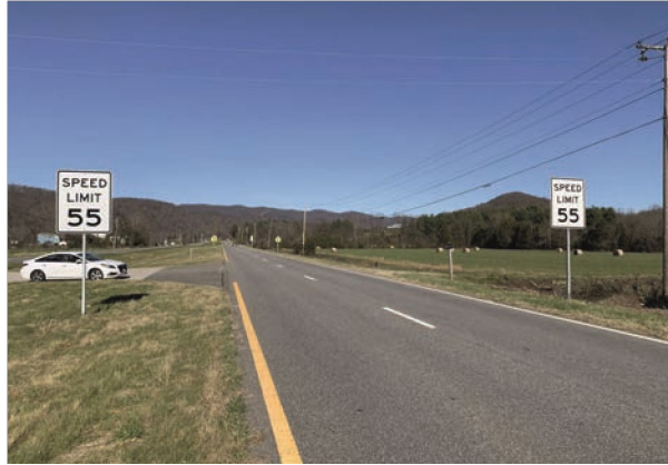
Figure 11. Photo. Conspicuity treatment: white retroreflective strip on signpost.
