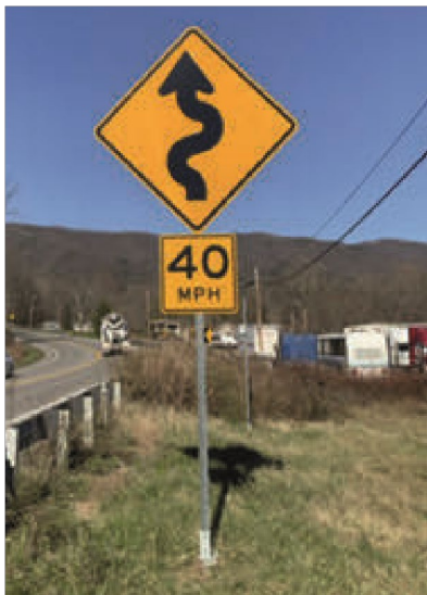
Figure 6. Photo. After treatment: oversized sign.
