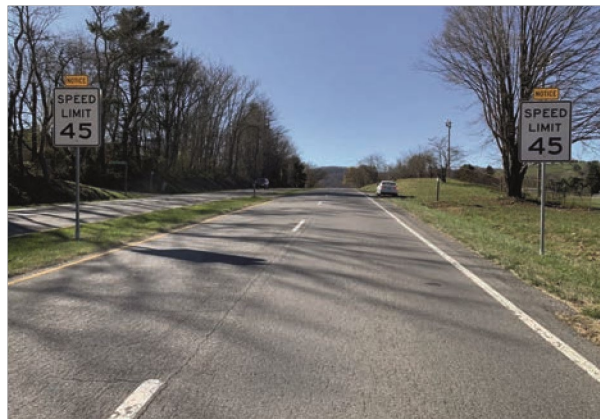
Figure 10. Photo. Conspicuity treatment : fluorescent yellow NOTICE header panels.
