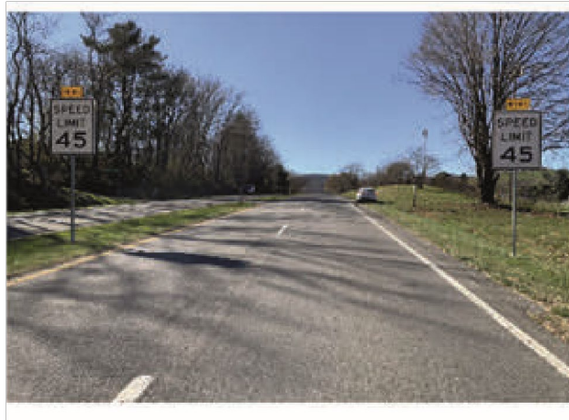
Figure 8. Photo. After treatment: fluorescent yellow NOTICE header panel.
