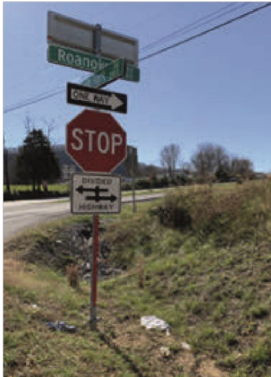
Figure 7. Photo. After treatment: red retroreflective strip.
