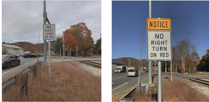
Figure 3. Photo. Before and After treatment: header panel.
