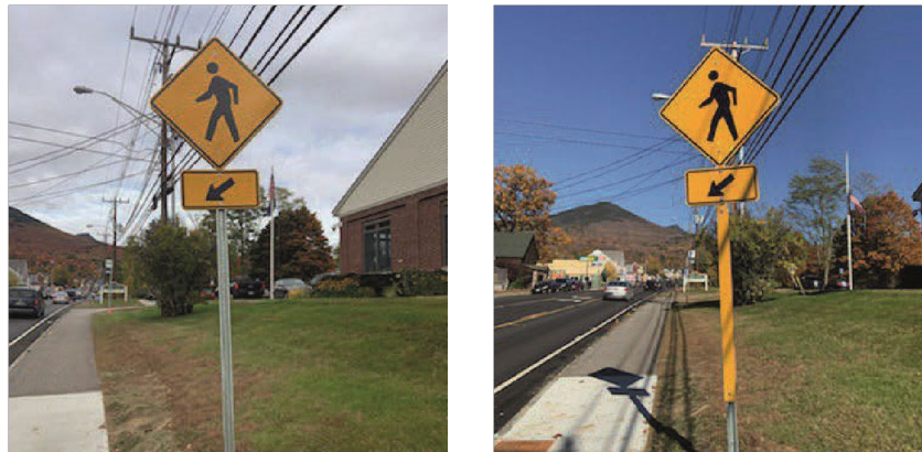
Figure 2. Photo. Before and After treatment: retroreflective 2.5-inch yellow strip.
