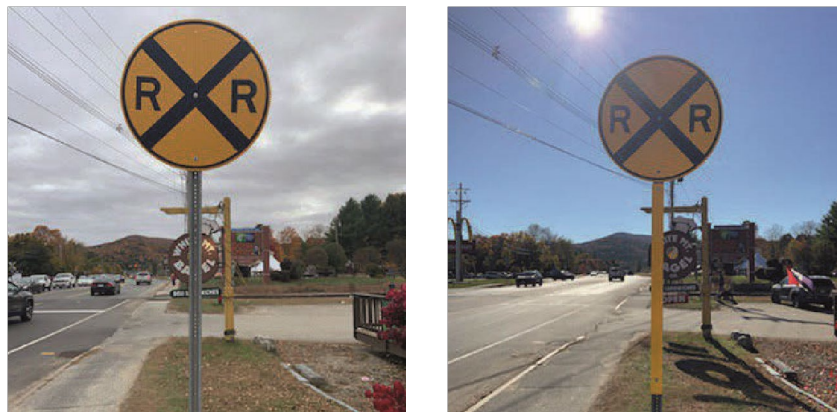
Figure 5. Photo. Before and After treatment: retroreflective 2.5-inch yellow strip.
