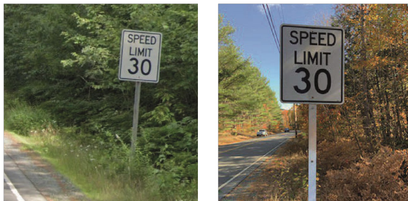
Figure 4. Photo. Before and After treatment: retroreflective white strip.
