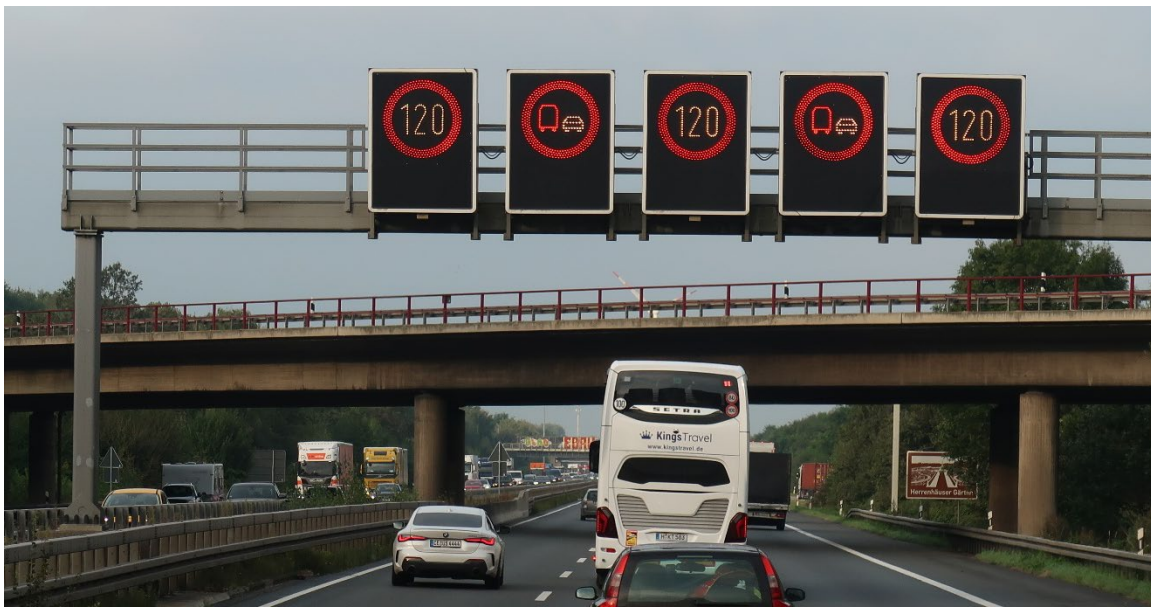
11 12 Figure 6 Changeable message sign on the Autobahn in Germany, entering a 13 restricted speed zone; the standard symbol sign conveys the meaning 14 that trucks are prohibited from occupying the left lane. 15
