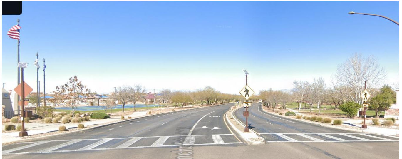
BEFORE: RRFB Crossing installation (cost $15,558 in 2024 dollars) excluding poles and foundations
