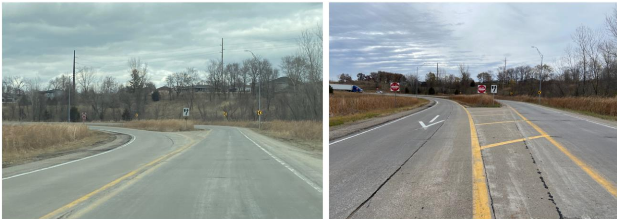
Figure 3. Same location showing before and after, where the standard Parclo B signage is shown on the left and the enhanced gateway treatment is shown on the right.
