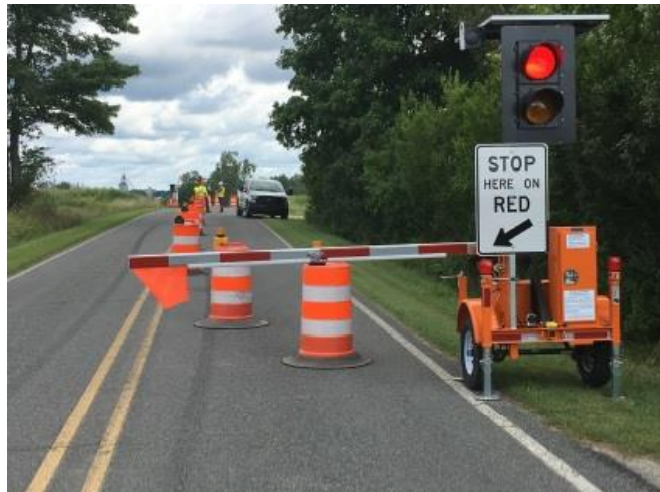
Figure 1. Closed Lane AFAD Application in Michigan (Image Courtesy Michigan Department of Transportation)
