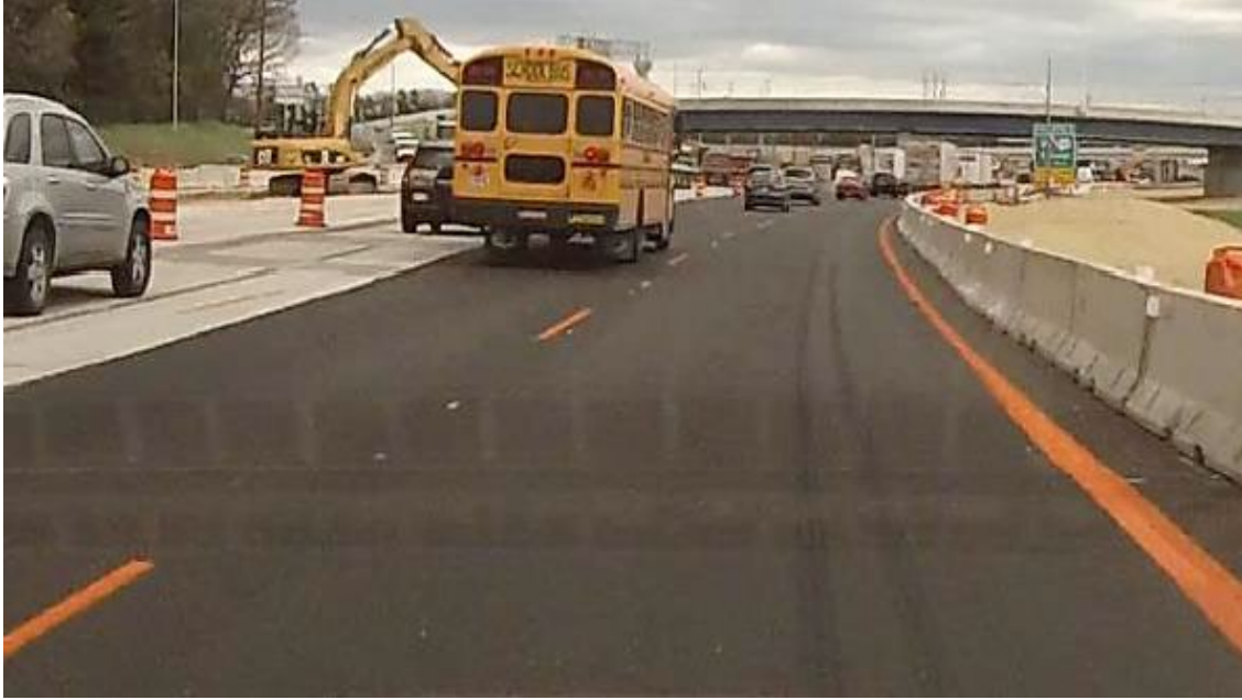
Figure 1. Orange Temporary Marking on Asphalt Surface
